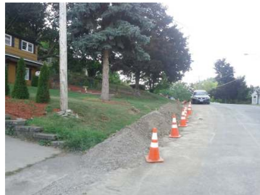
Fig 4 Residential Test Area with gas construction
