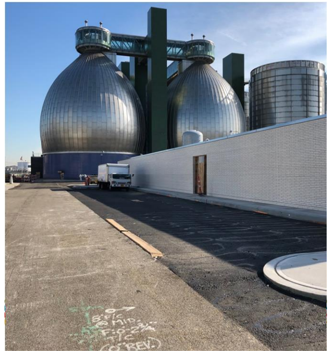
Digestors at Newtown Creek Wastewater Treatment Plant and location of the NYSEARCH Living Lab beyond the walled area
