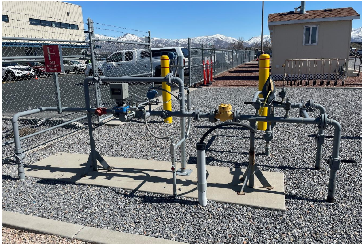
Dominion Utah showcased a hydrogen injection system at the NYSEARCH Quarterly March meeting in Salt Lake City, UT. The system is made up of specially designed metering, gas quality, and odorization equipment to deliver 5% vol hydrogen into Dominion's distribution system.
