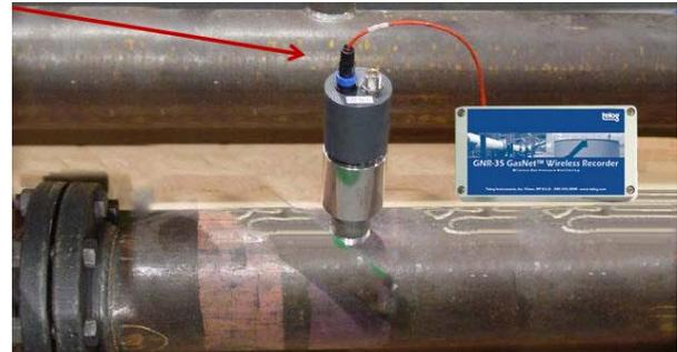
Figure 1: GasComm<sup>TM</sup> installed in Steel Pipe
